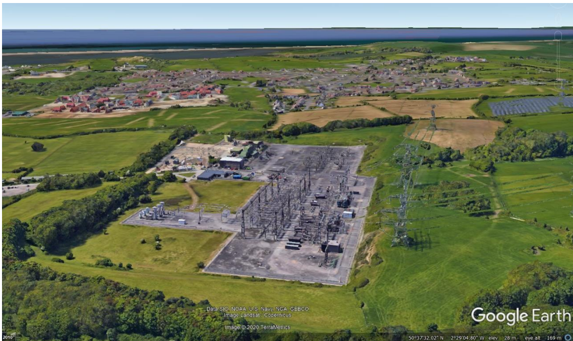
Plate 4 - Aerial image of Chickerell Substation
