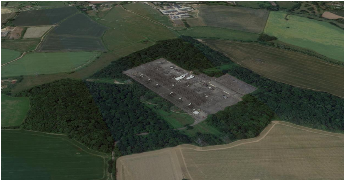
Plate 6 – Aerial image of Bramley Substation
