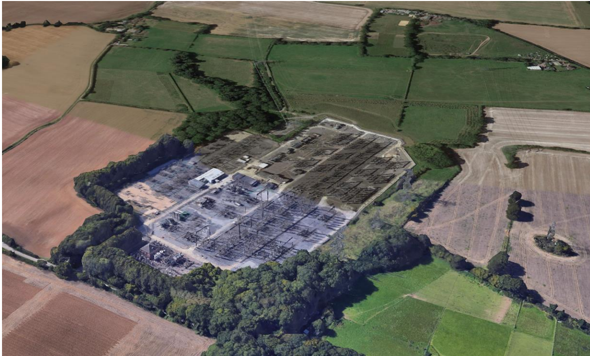
Plate 7 – Aerial image of Lovedean Substation
