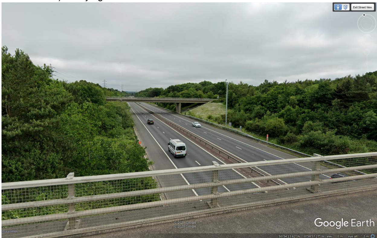
Plate 16 - Street view of 1D-HDD10 Crossing B2149 and A3 (M) roundabout
